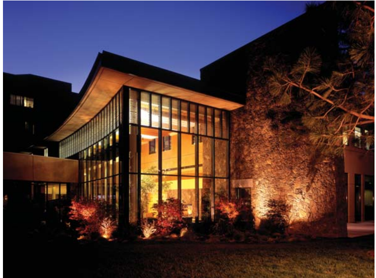
ACOUSTICAL DESIGN OF THE FAMILY BIRTHING CENTER AT SAINT CHARLES MEDICAL CENTER IN BEND, ORE., INCLUDED ACOUSTICAL SEPARATION BETWEEN AND AROUND THE ROOMS OF THE NEONATAL INTENSIVE-CARE UNIT. PHOTO CREDIT: CALLISON ARCHITECTURE/CHRIS EDEN.
